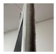
• Now repeat with the second screen but this time put the pile to the back of the frame i.e. closest edge to your door frame.
